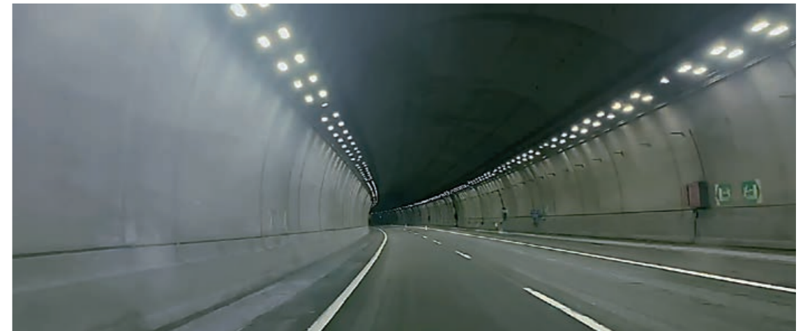
Lantueno Tunnel, A-67 Highway - Santiurde de Reinosa, Spain
